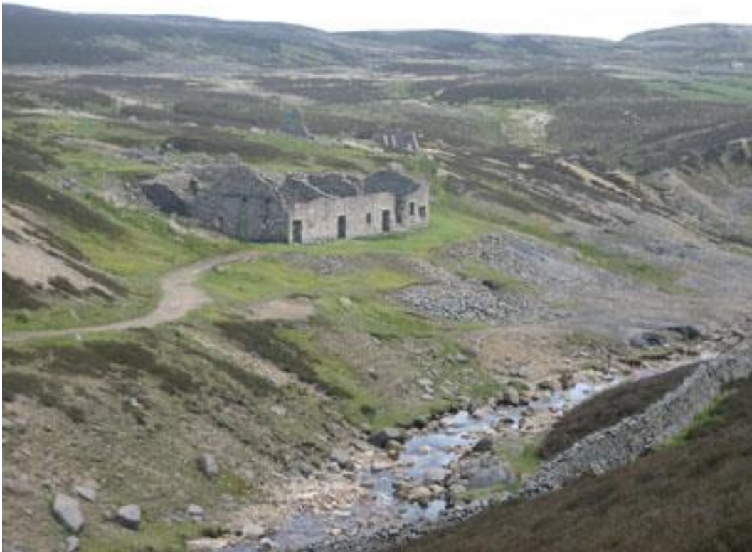
Swaledale lead mines. Photo by Author 2007
