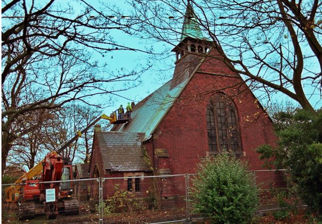
Figure 13. Removing the roof slates (looking from west wall of chapel).
