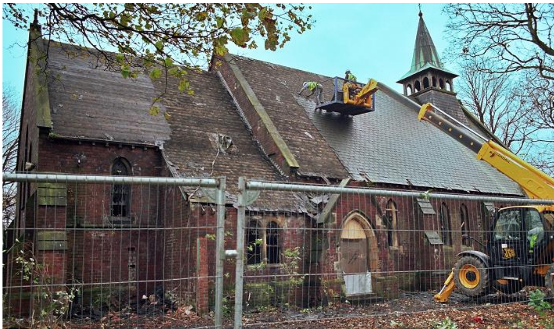
Figure 14. Removing the roof slates (looking from north wall).
